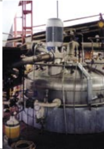
Defoamer 600P mounted on production-fermenter for biopolymers
